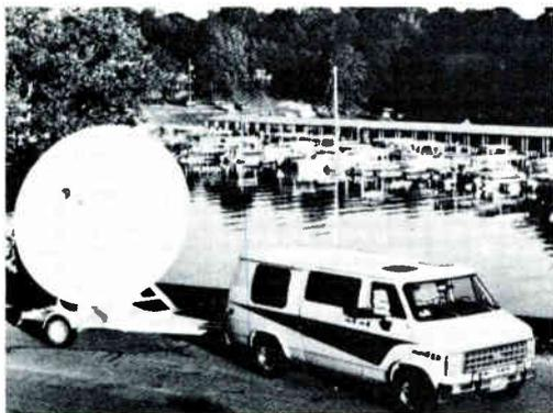
**A SUPER TVRO ANTENNA SYSTEM.** High-quality panelized aluminum 11-foot dish and steel polar mount. Dish weighs approximately 200 pounds, mount 265 pounds. Precision designed, easy installation, zinc chromate base primed and heavy-duty white top finish. The rotating feed is standard! Easily shipped and installed. Choice openings for dealers and distributors.
