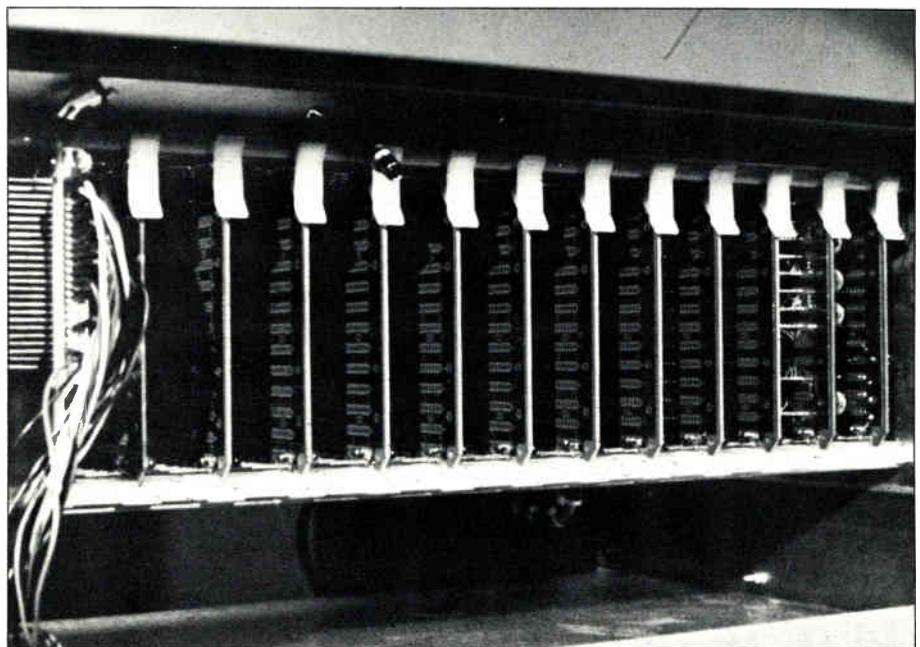
Figure 8 Front of I/O expansion unit card cage—note clearance below cards for cables
