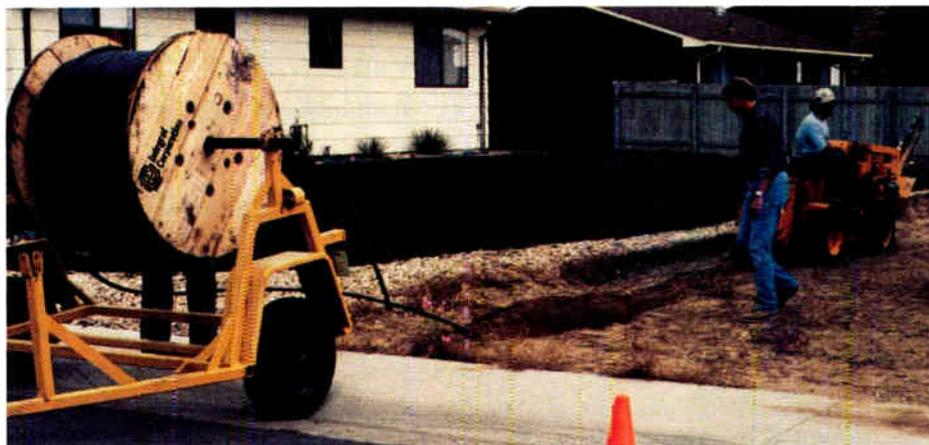
Coax-Cablecon makes for a fast installation: it arrives at your job site on reels, pre-cut to 1200 or 2400-foot lengths. Small back-lot tractors can plow-in Coax-Cablecon up to 60% faster than other in-duct buried systems: in-field demonstrations have averaged 60-feet per minute in medium density soils.
