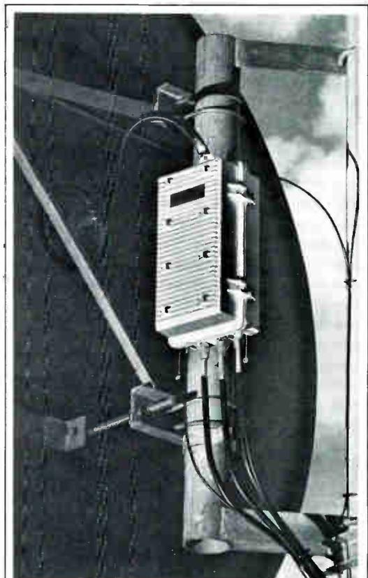
Micro-Beam<sup>™</sup> transmits up to 60 channels from a simple tower-mounted unit—no air-conditioned buildings, extensive waveguide or expensive klystron amps.
