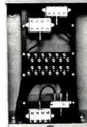
CWY's Omni-Rack™ system uses rails and panels similar to headend rack accessories to take the tangle out of multiple dwelling enclosures. This money- and time- saving system easily adapts to fit existing installations and is versatile enough to conform to your own design.
