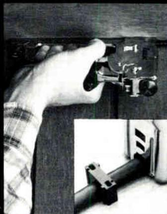
It's easy to use. The Fastac Clip Gun and its companion RB-2 Cable Clips will install drop cable on any wooden surface solidly, quickly, and flawlessly. It's error free. Installations proceed smoothly and trouble calls resulting from cable damage are eliminated.
