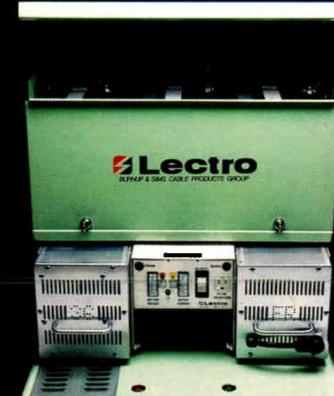
Sentry II simplicity also means that maintenance takes only minutes. Because Sentry II is the only standby power source with modular plug-in design, the only service tool you need is a key to open the cabinet, then slide one module out and simply plug a new module in. So it not only reduces service costs, but helps to ensure customer satisfaction and subscriber retention.
