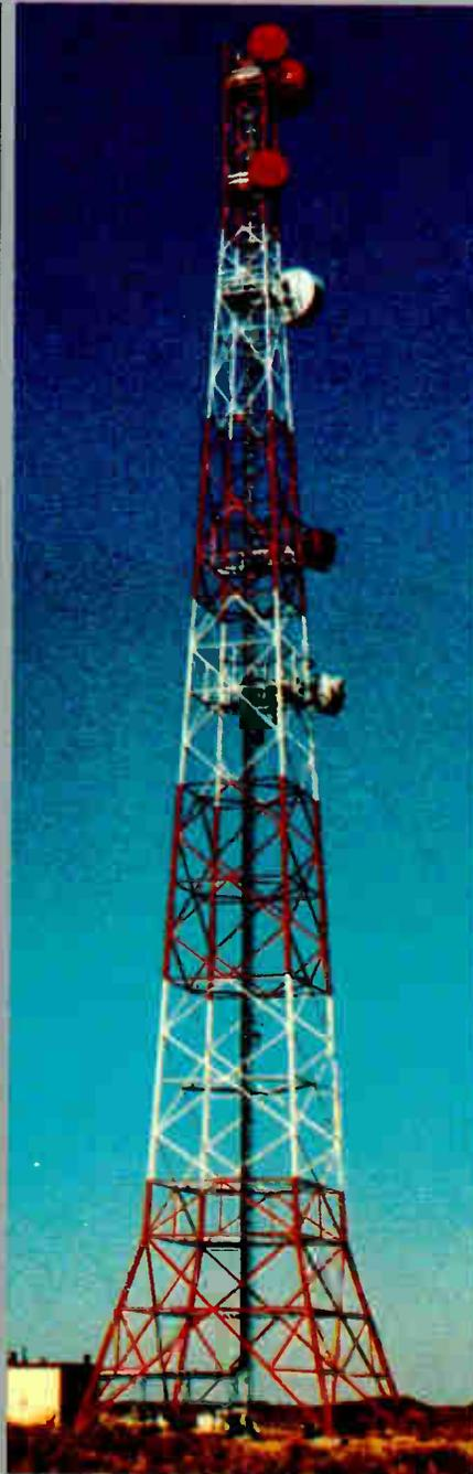
Microflect's 800 Series towers are available in heights from 5' to over 400'. Flexibility, in terms of capacity, framing options, and future load capabilities, is a major design consideration.
