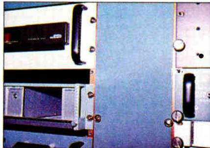
*A 7-inch wide copper strip is installed from rack to rack*
