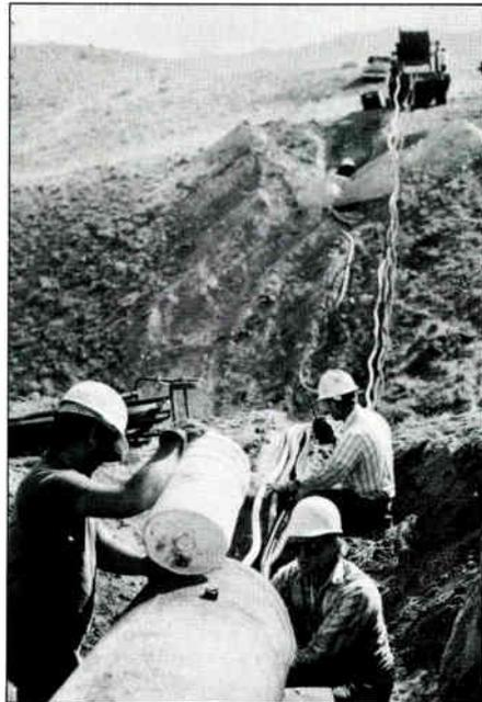
*Vyvx's NVM system being installed through decommissioned pipelines*
