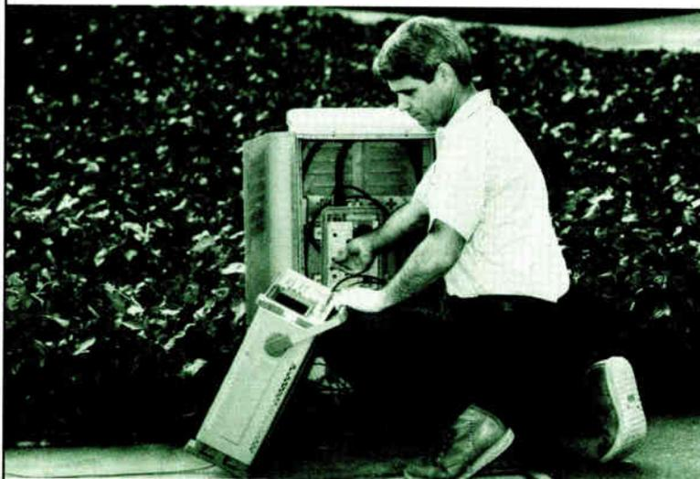
**HP's portable CATV analyzer speeds up troubleshooting.**
