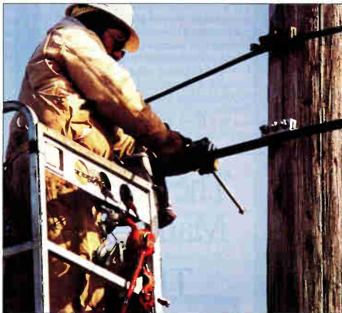
*New messengered duct installs easily.*
