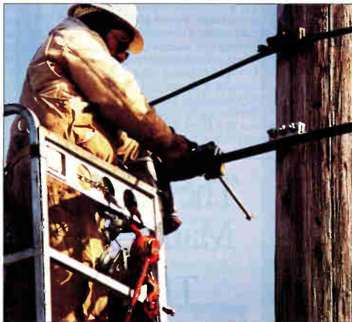
*New messengered duct installs easily.*
