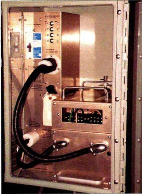
*Interior view of the pole-mounted power node designed by Comm/Net Systems. It shows the dead-front design along with the removable transformer module and circuit breakers.*
