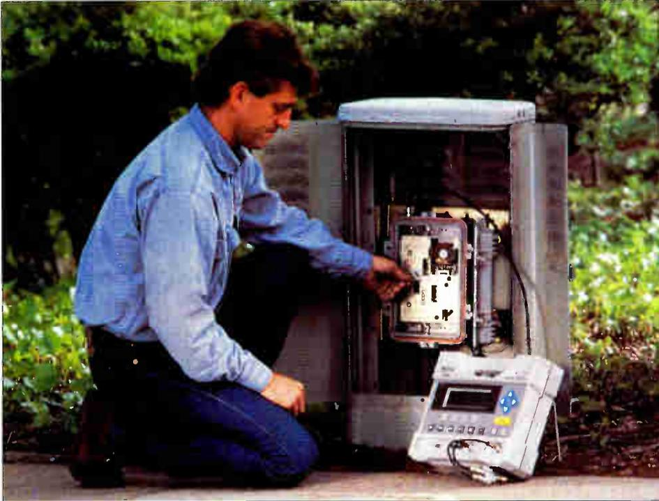
*Return path alignment using the HP CaLan Sweep/Ingress Analyzer.*
