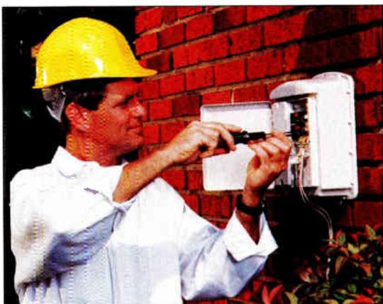
Scientific-Atlanta’s CoAxiom Customer Interface Unit can be powered from the network, or locally powered from the subscriber.
