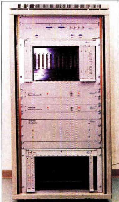
*In the headend, GADline features a management interface unit, frequency transverter and convertor units, a splitter combiner and a trunk interface unit.*
