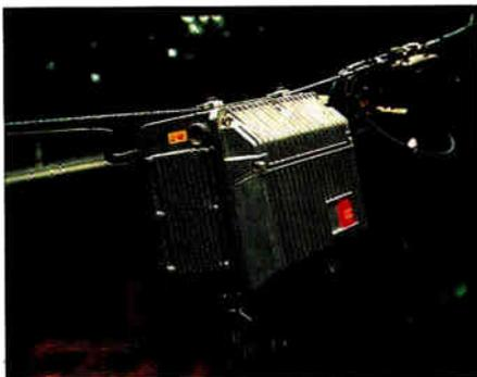
ADC’s Multi-Dwelling Integrated Services Unit features configurations ranging from 12 to 96 lines and provides remote provisioning of both video and telephony services.
