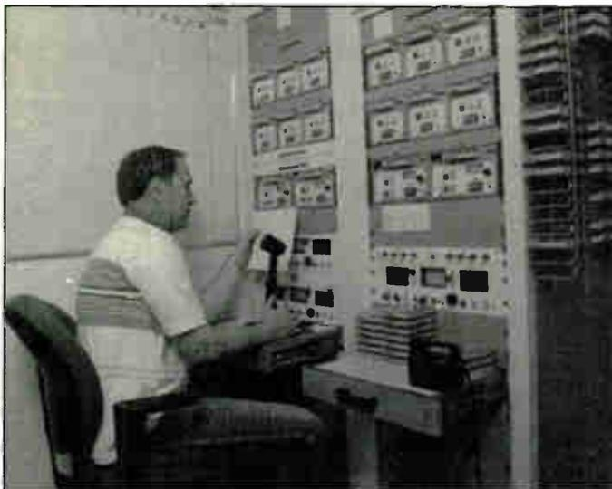
*National Weather Service offices throughout the country make regular broadcasts of weather forecasts and severe weather watches and warnings over NOAA Weather Radio transmitters using frequencies between 162.4 and 162.55 MHz. Many of today's CBs are specially-equipped to monitor such broadcasts.*
