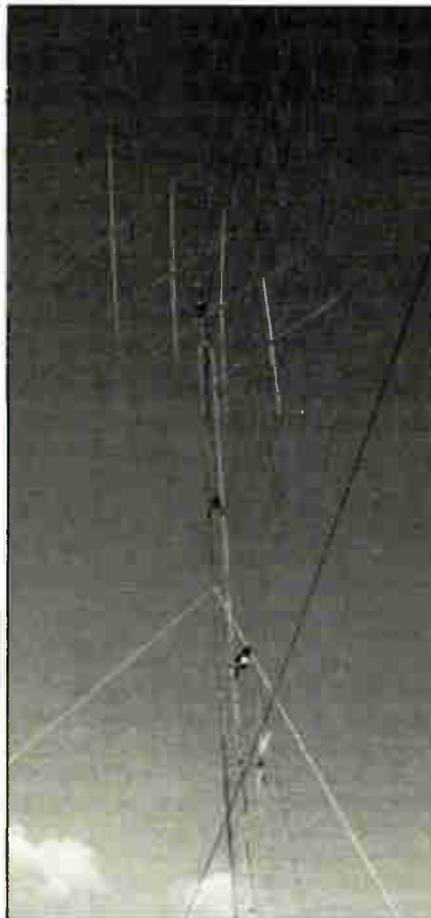
Unlike this operator, you should always remember to mount your rotor INSIDE the tower and use a thrust bearing to minimize bending movement.
