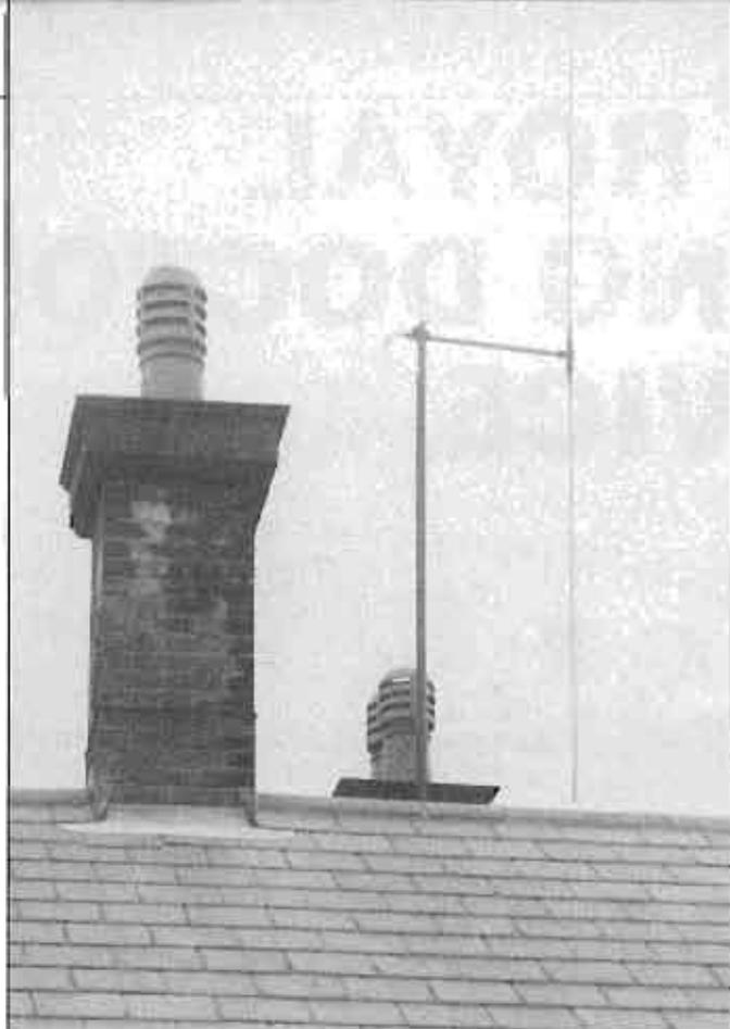
Antenna mounted on top of hospital complex (vertical dipole, centre fed).
