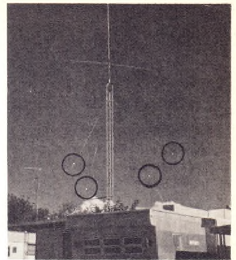
Reduce TVI caused by re-radiating guy wires. Install strain insulators every three feet.
