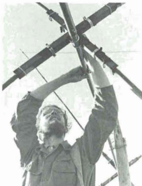
*Step 6*— Fastening the wire to the cross-arms. First, you'll need to cut a piece of wire to make each element out of. Cut the following lengths of wire: 38'2"—reflector; 34'10"—driven; 31'4"—director. Remember to keep it straight where each wire goes so as to get the right length of wire on the right set of cross-arms — IT'S IMPORTANT!
