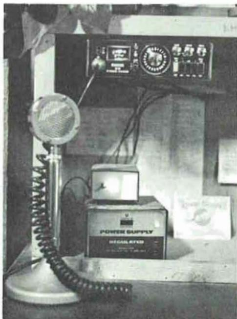
**Hooking up the car battery and charger:** It should be located within fifteen feet or so from the radio, so you don't lose too much juice running long wires.
