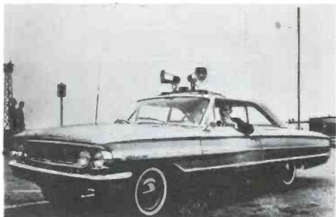
North Tripp Ave., Chicago, Ill. 60646. The 32-watt, all transistor, system plugs into the cigarette lighter of your 12-volt car. Inputs are provided for both microphones and radio/phonographs, and outputs for 8 and 16 ohms. Two speakers and mounting bracket are supplied, as well as a noise cancelling mike. Price of the complete sys-
