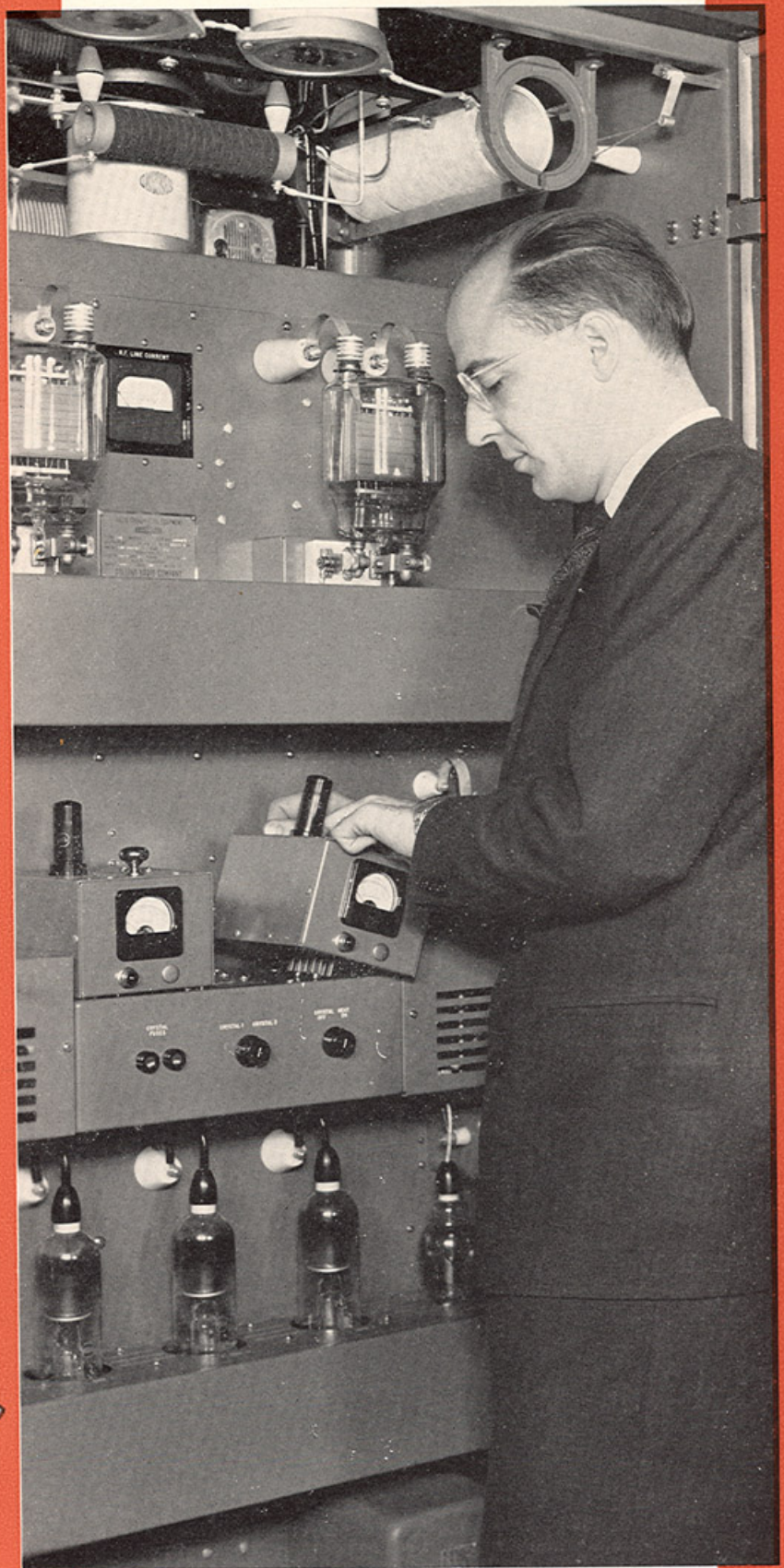
Either oscillator unit can be removed quickly. The selector switch is set to the second unit and transmitter operation continued while the removed oscillator is checked.
