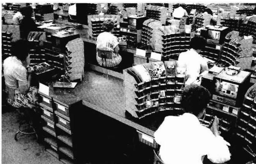
Production areas in Building 106 featured "teleguides" in front of assembly operators to give detailed assembly instructions via an audio-visual presentation. 1961 photo.
