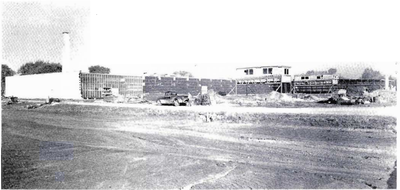
Above Floor space of the Main Plant was doubled during the fall of 1941 when additions were built on the south and east sides. This view faces northwest.
