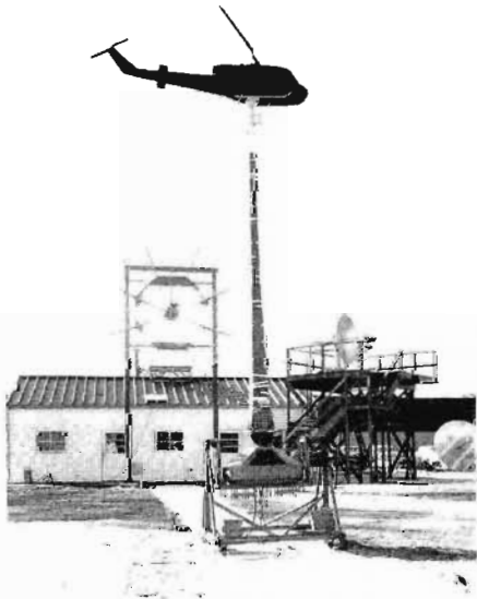
Special support towers held and rotated aircraft models for measurements on antennas mounted on the model aircraft. The height provided a free space effect. 1959 photo.
