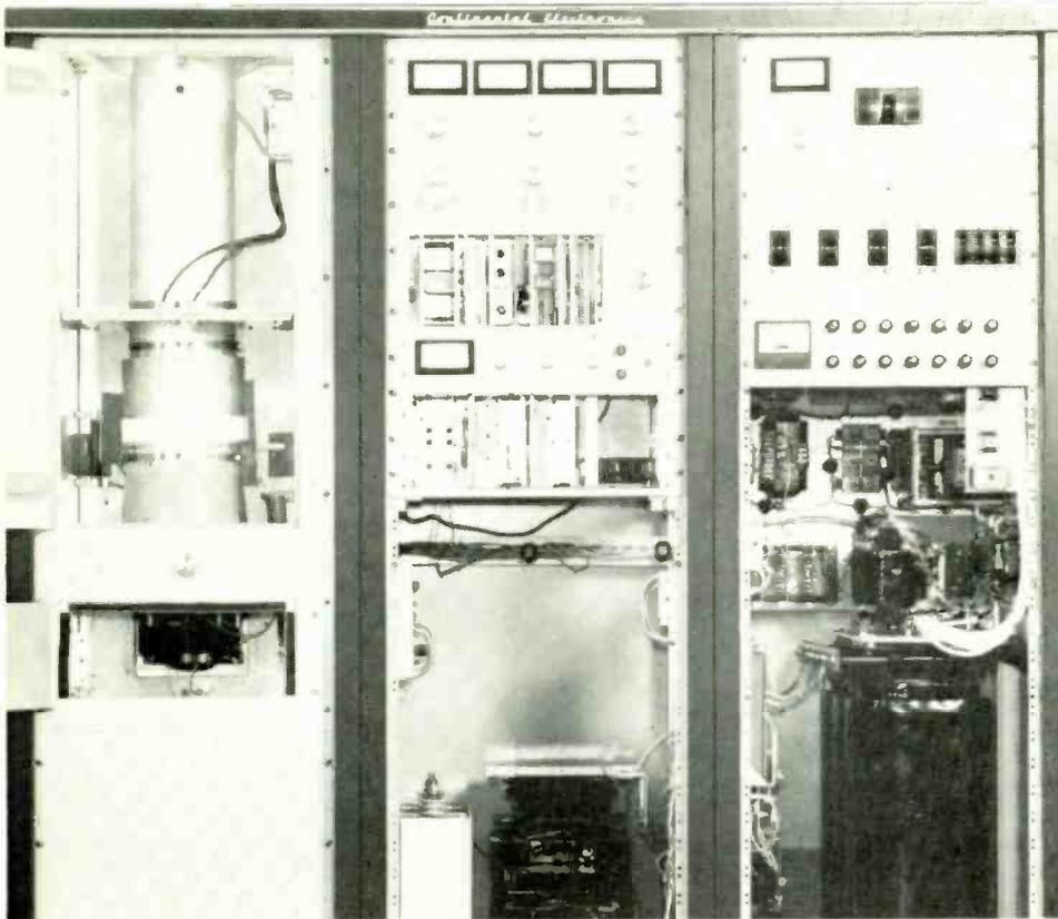
grounded screen tetrode design eliminates screen bypass capacitors and provides excellent stability.
