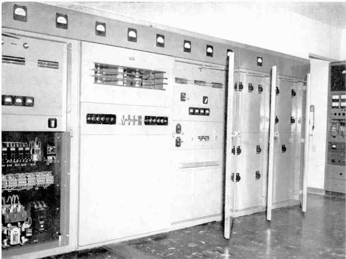
Below—Gates BC-5B 5000 watt equipment with five tower phasing equipment in matching cabinet at WENE, Endicott, N. Y.
