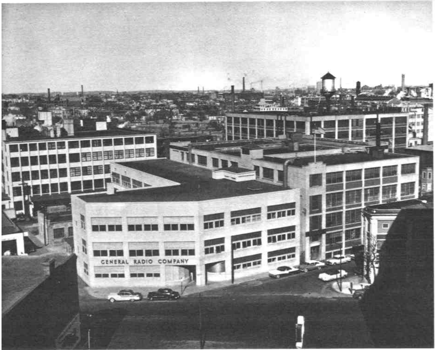
General Radio's final Cambridge plant. Building in foreground, a converted garage, housed administrative, engineering, and sales offices.
