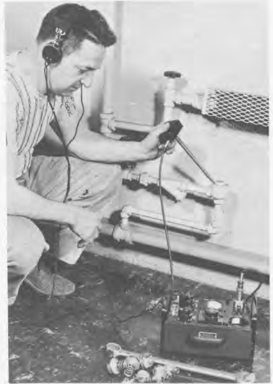
Figure 36. Checking a steam trap with vibration-measuring equipment.
