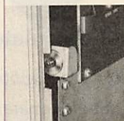
Safety interlock switch guards against shock hazards.
