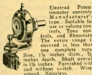
Electrad Potentiometer controls, Manufacturer's type. Suitable for use as volume controls, Tone controls, and Rheostats. The entire range is covered in less than one complete turn.
