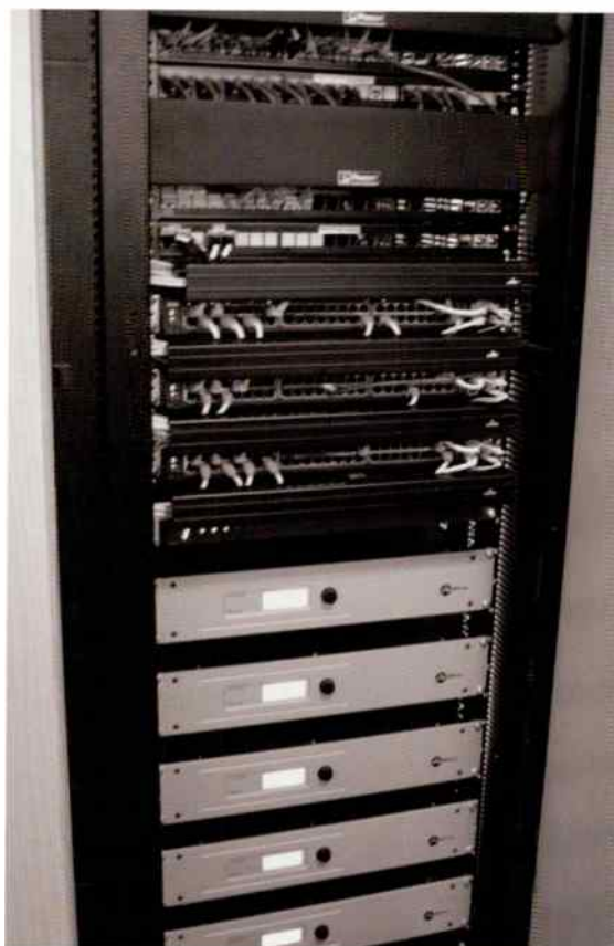
Neat high-density Ethernet and Axia DSP mixing engines power MPR studios
