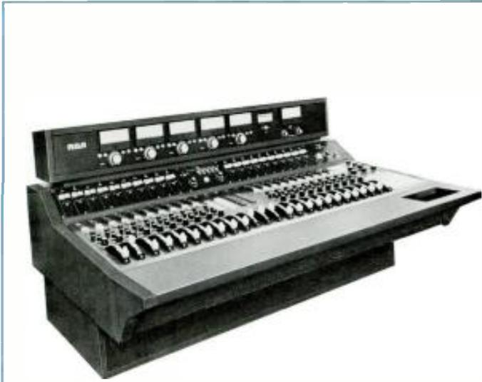
Built especially for Lewron Television in New York City, this is one of two custom audio consoles recently installed. The console offers 20 inputs, which accept either high- or low-level signals, fed to any or all of four output channels. A fifth output channel is equipped with built-in AGC. Each output channel feeds a one-by-two splitter. Also included is a slating switch and a built-in tone oscillator.
