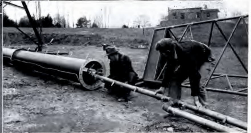
Inserting the transmission line harness into the two-section Pylon at WSBA-FM, York, Pa.
