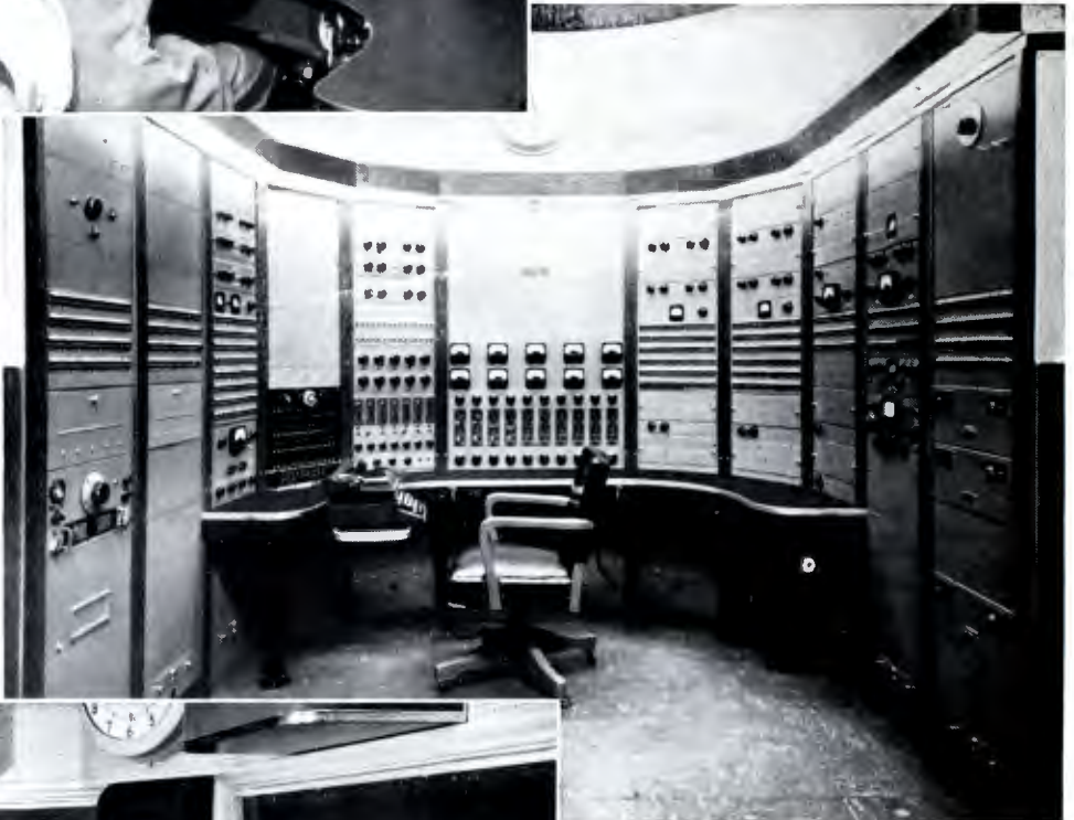
WNEW, New York. This master control installation in WNEW's 7-studio lineup is flanked on each side by 5 deluxe audio equipment racks. It has complete facilities for control and preset switching of 7 studios to 10 outgoing lines . . . and for feeding cue from any channel to any studio.
