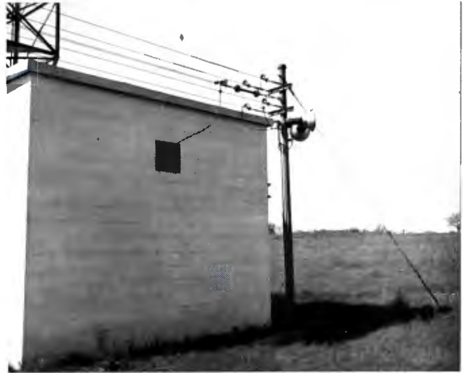
Typical installation of MI-28012-A Dead-end Kit (using pole)
