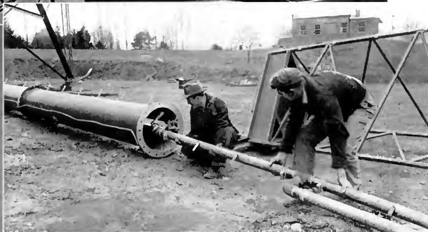
Inserting the transmission line harness into the two-section Pylon at WSBA-FM, York, Pa.
