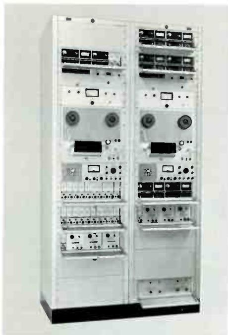
Two of the many racks of Audio Equipment for Station KRON are seen here, they contain cartridge and reel tape audio recorders, latest style BA-40 series amplifiers, and other solid-state audio components.
