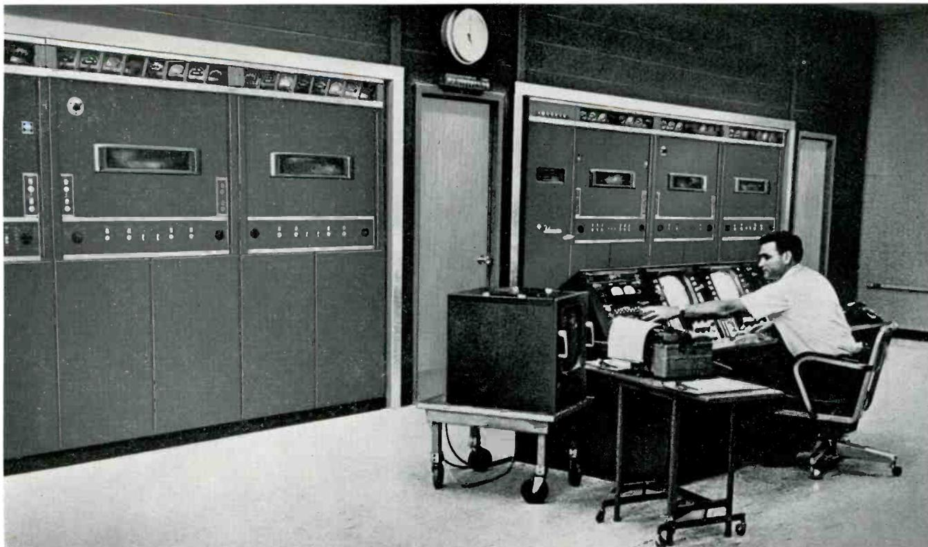
TT-50DH Transmitter installation showing the two 25-kw transmitters and control console employed by Station WNAC-TV, Boston, Mass. This is the first parallel television system in the United States.
