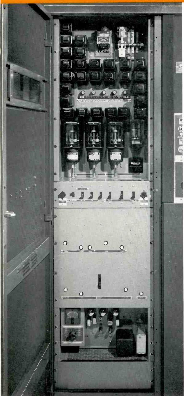
Control cabinet with door open showing auxiliary switches, breakers, overload and auxiliary relays. Overload indicating lights for all TT-25DL circuits are grouped on strip that can be seen through window when door is closed.
