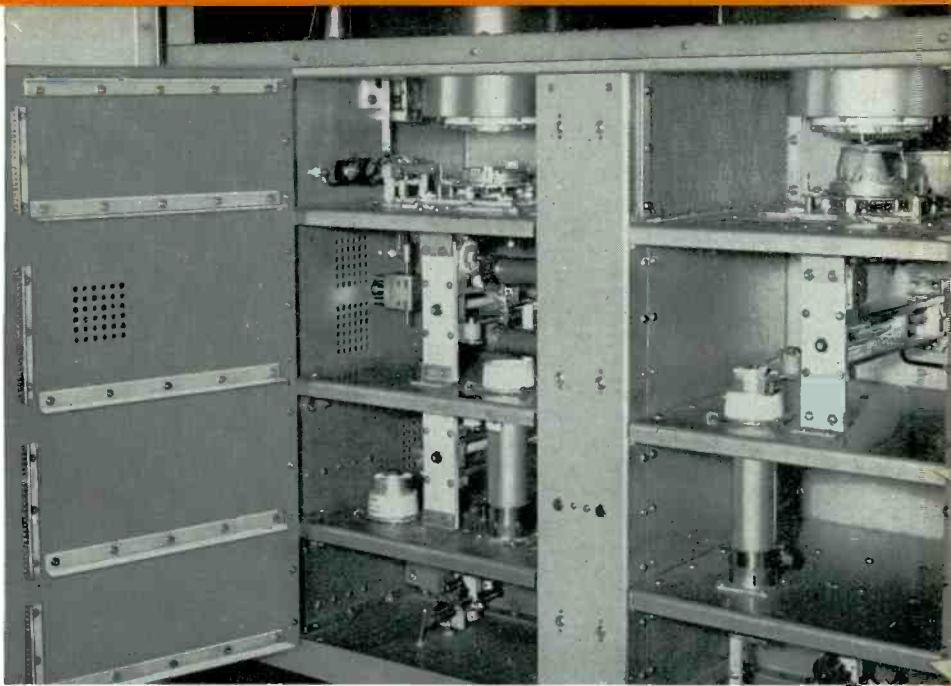
existing buildings. Reduction of required floor space is effected by the walk-in enclosure design of the TT-25DH.
