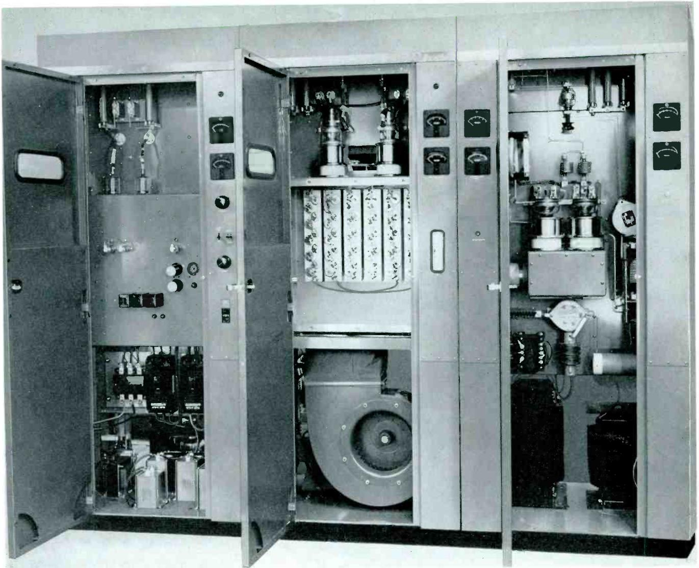
Type BTA-10U 10-KW AM Transmitter showing front view of driver-control, Modulator and High Voltage Rectifier, and power amplifier cabinets.
