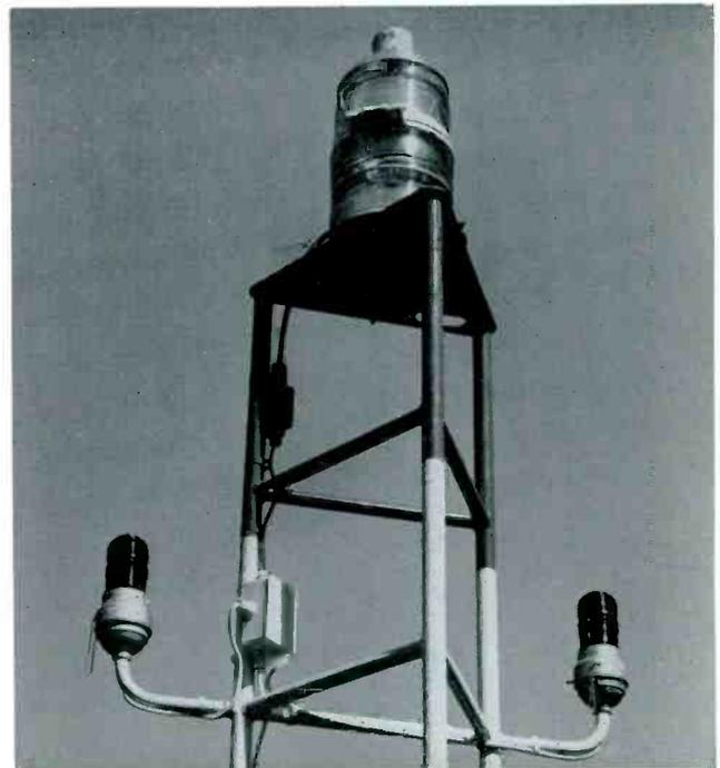
Main beacon and side obstruction lights shown powered by use of either lighting transformer or lighting choke coil.
