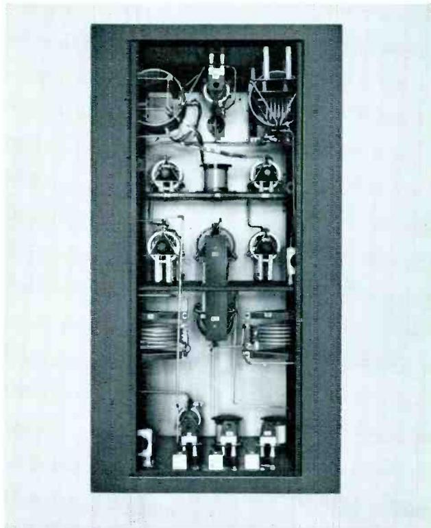
Phasing Cabinet showing simplicity of design and layout. Custom equipment provides maximum stability for dependable AM operation, for three tower, 10-KW stations.
