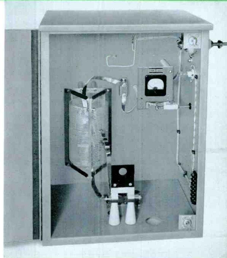
Basic 1 KW Antenna Tuning Unit, MI-27767-A.
