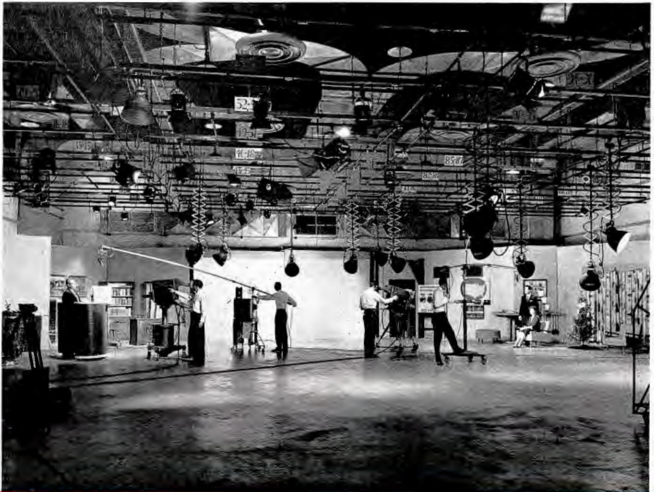
General view of a studio showing flexible lighting arrangement which provides "third-dimensional" effect, head-on, or general illumination as required for various sets.
