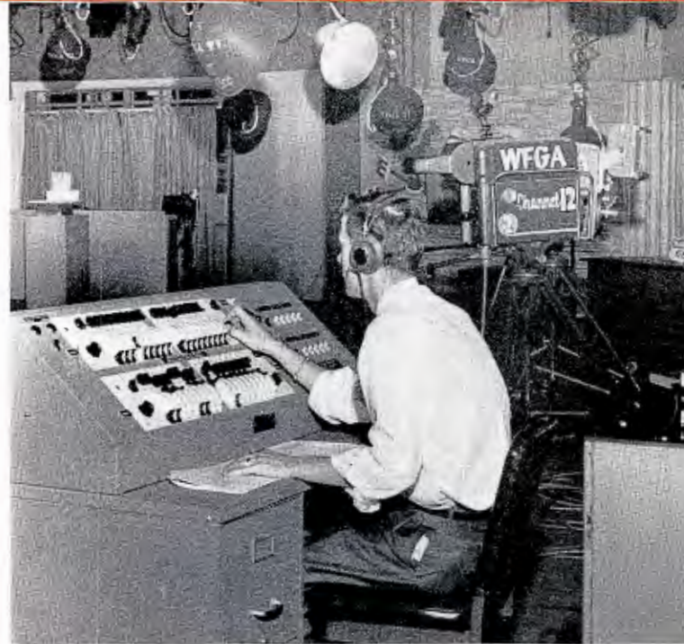
View of studio at Station WFGA-TV, Jacksonville, Fla., with electronic dimmer lighting control and patchboard in extreme right corner.
