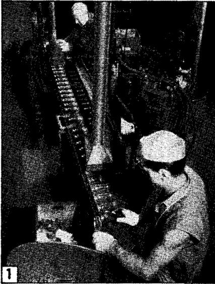
(1) *Carbonizing interior walls of glass bulbs*—This machine places a band of carbon dust within the bulb—then neatly cleans the top and bottom section of the bulb.
