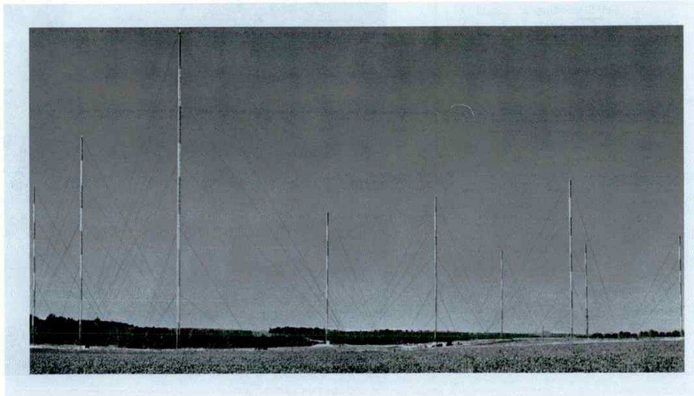
area on all flat surfaces and 20 pounds on round surfaces. This is the equivalent of an actual wind velocity of 86.6 mi/h (139 km/h). Towers with higher wind-load ratings are, of course, available. Towers are designed in accordance with EIA specifications RS-222B.
