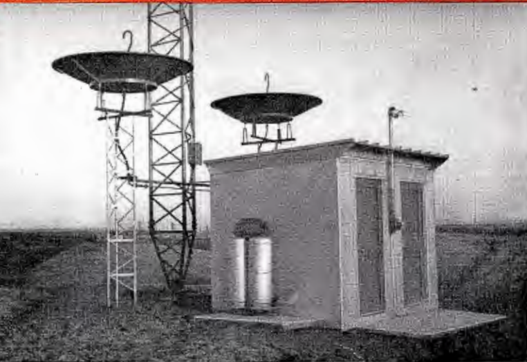
RCA parabolic reflectors shown at a typical microwave repeater station.
