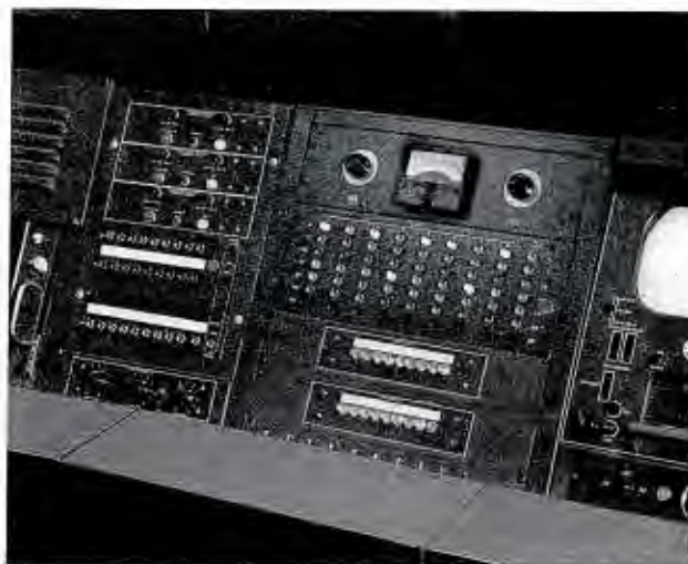
View of the television tape switching control panel at master control in Reeves Sound Studios. The inputs to six RCA Tape Machines are all switchable at this central location.
