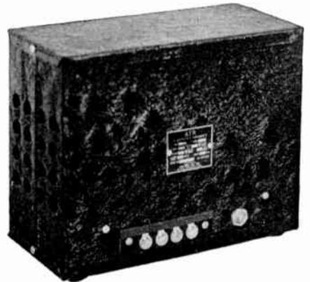
Illustrating ATR Vibrator Pack complete with audio filter, Style B.
