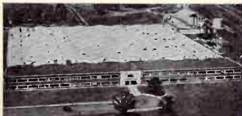
Westinghouse at Elmira, N. Y. 360,000 square foot picture tube plant and division headquarters.
