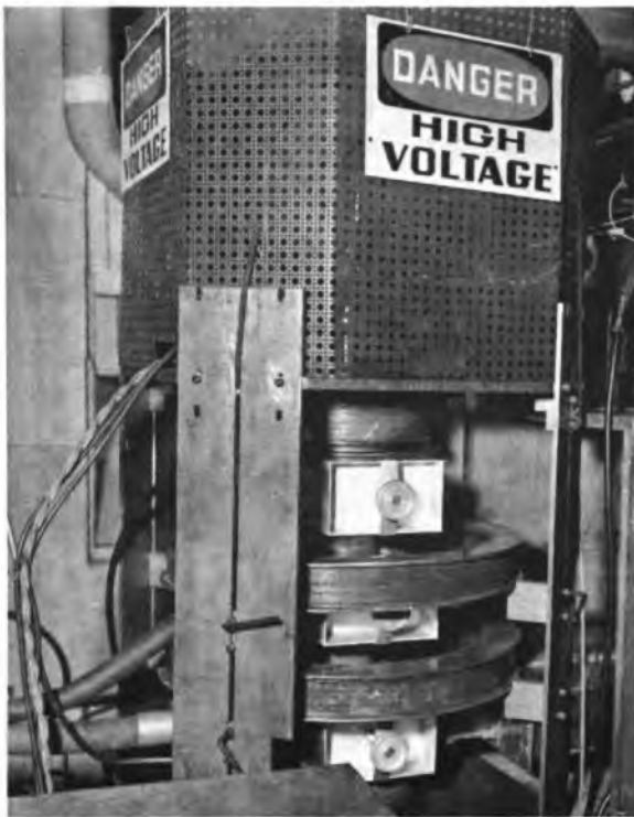
Fig. 8—The 5-kw klystron on test.
