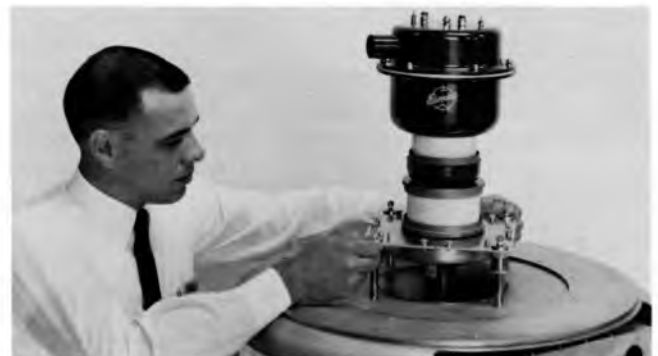
Figure 16—Adjustment of Prefocus Coil.
