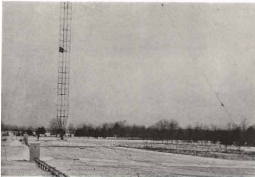
View of nitrogen filled coaxial transmission line and 650-foot Blaw-Knox radiator.
