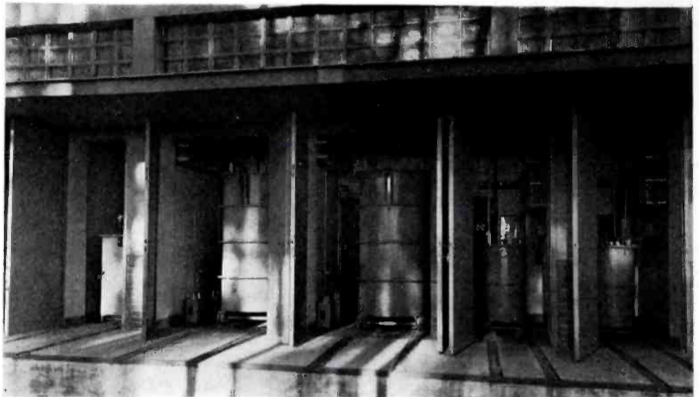
View of audio-frequency transformer and reactor cubicles, showing one of the five reactors, the two modulation transformers, and the two interstage transformers. Among the unique features of this transmitter is the provision for cutting in quickly the complete reserve equipment. This is done by employing cubicle construction and by placing the reserve equipment on tracks so that it can be moved into place quickly.
