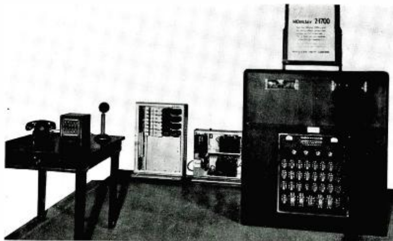
Fig. 6. The J. L. Franklin Automatic Time Telling installation. Note the emergency hand set equipment at the left. The time devices are mounted atop the large cabinet at the right.
