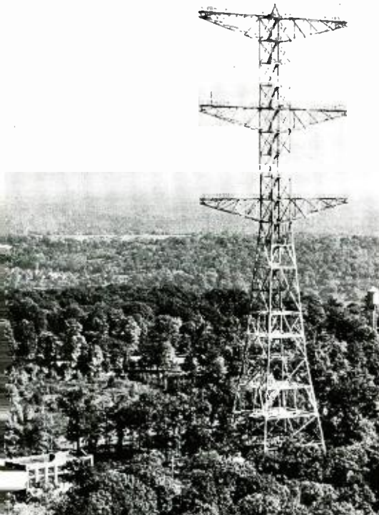
Fig. 4. First 50-kw u-h-f f-m transmitter—W2XMN, Alpine, N. J. (near N. Y. C.). Designed, constructed, operated by Major Armstrong.
