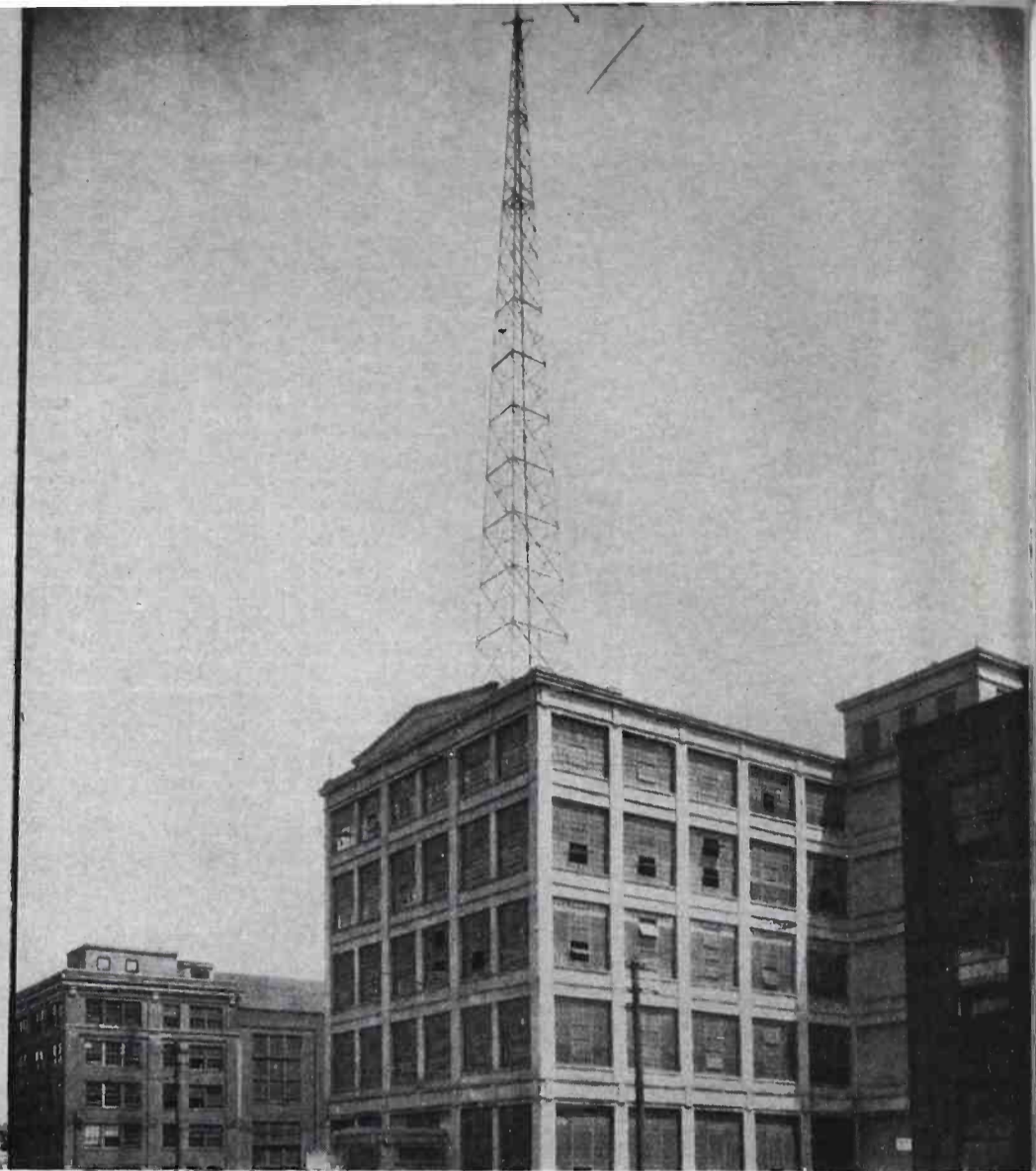
One of the pairs of towers for WGY's first transmitter in 1922.
