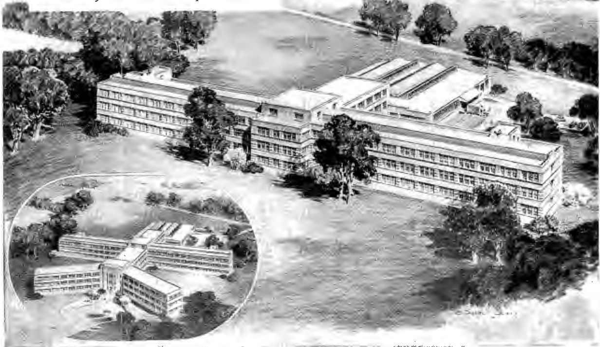
Main section of the new RCA Laboratories under construction at Princeton, N. J. This section will open in 1942. Inset shows the Laboratories as they will look when completed.
