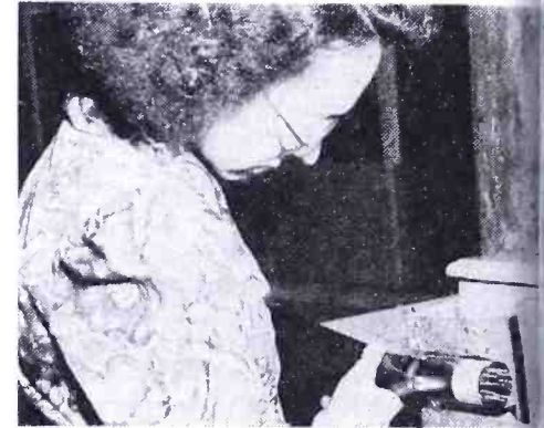
Figures 13 (above) and 14 (below) Figure 13, flashing the getter by high frequency after the tube has been pumped and has had its base attached. Figure 14 checking electrical characteristics and light output on cathode-ray tubes. Preheater at lower right makes preliminary test for short and voltage breakdown.
